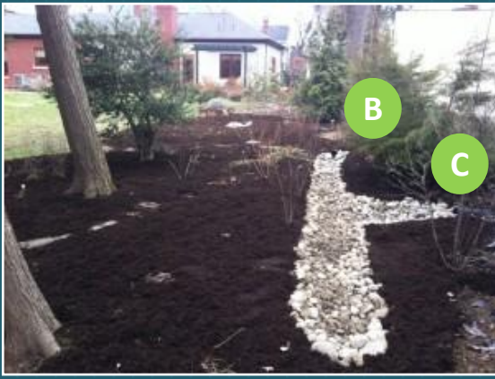
Dry creek capturing rainwater runoff
